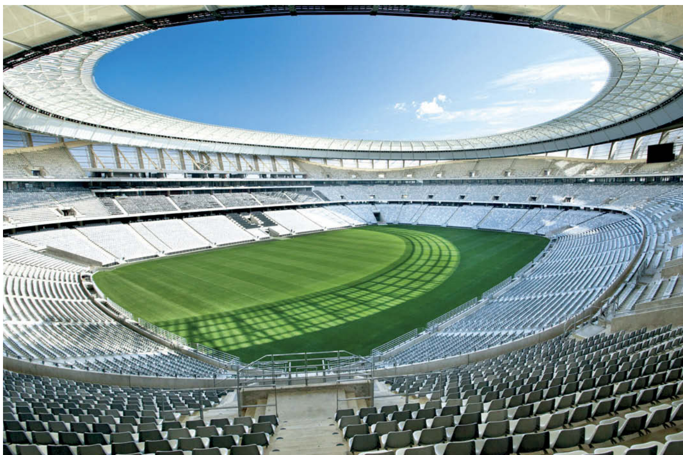
Greenpoint Stadium Republic, Africa de Sud. Forum Seating
