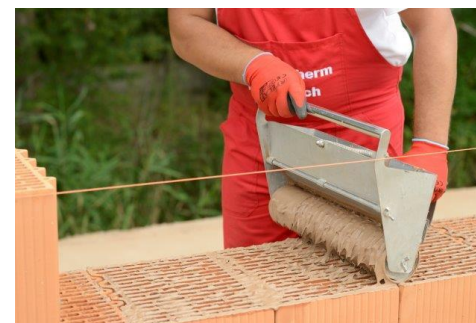
Aplicare mortar Porotherm Profi
